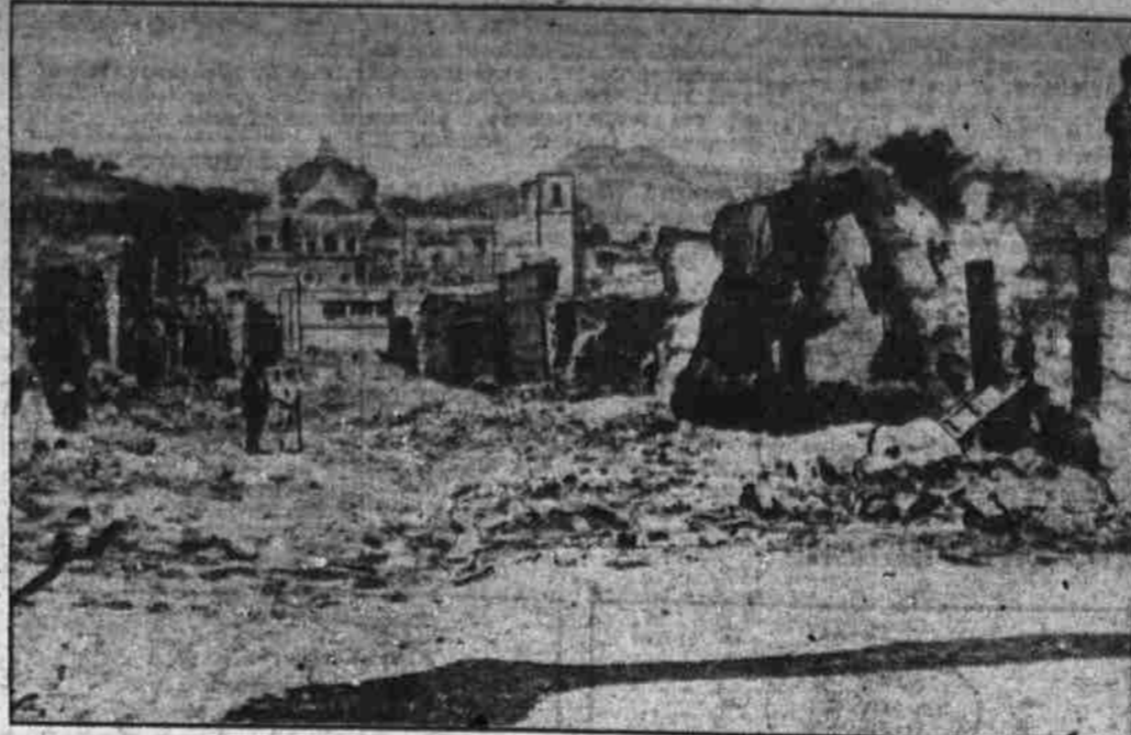
The city of Oaxaca, with most of its buildings in ruins, was one of the hardest hit in the recent earthquake in Mexico. Nearly 50 lives were lost. One of the streets lined with wreckage is shown here.
