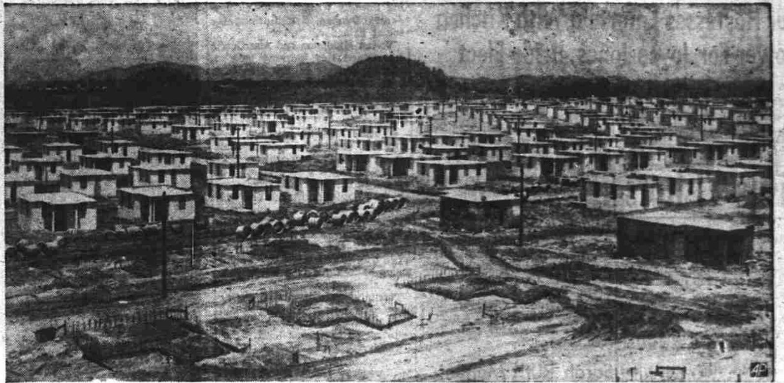
PUERTO RICO HOUSING PROJECT — These are part of 7,000 five-room concrete homes which are being built near San Juan, Puerto Rico, at the rate of 30 per day. They will sell for $4,000 with payments of $25 monthly. Non-veterans must put $400 down; veterans nothing. The Insular Government worked out $30,000,000 project with help of Leonard D. Long, Charleston, S.C.
