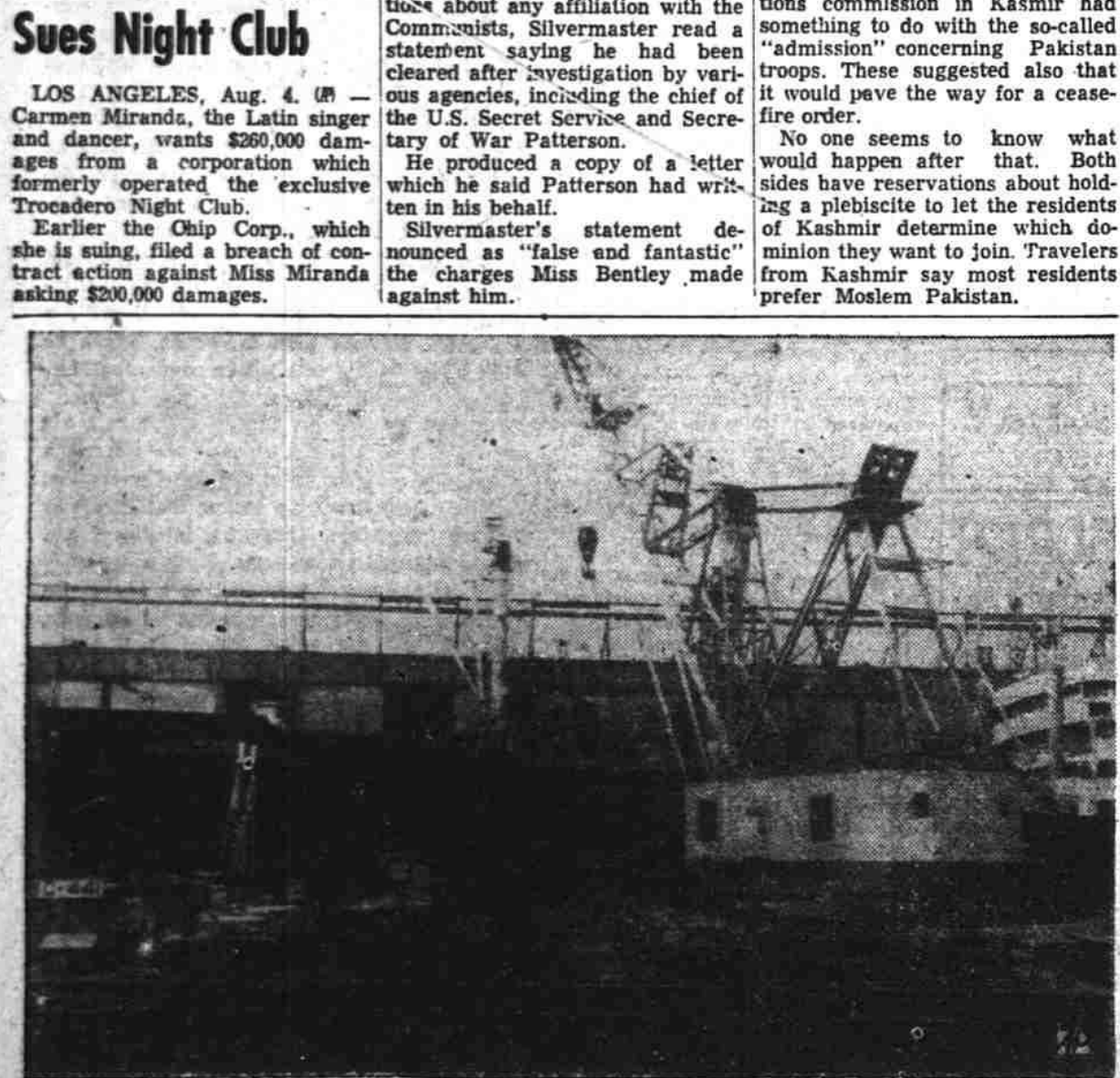
ORDNANCE EQUIPMENT EN ROUTE TO BRITISH ISLES. Cranes, trucks, tractors and other ordnance equipment, part of the first of several shipments to be sent to the British Isles, are loaded on the Army transport Oglethorpe Victory at Pier 12, Staten Island, New York City. (AP Wirephoto)
