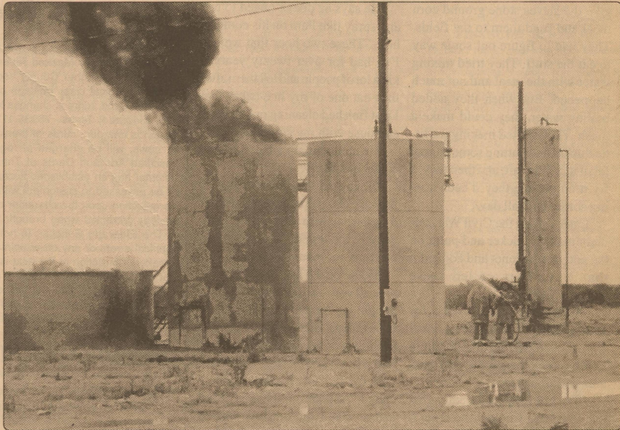
photo by Randy Mankin Blazing tank battery — The first firefighters on the scene at this tank battery fire Sunday, sprayed water on an adjoining tank to cool it down while awaiting for other units to arrive. The fire, believed to have been caused by lightning, occurred on Discovery Operating Company's "Box A #1" lease. In all, four units responded to the scene and the fire was quickly extinguished with foam.
