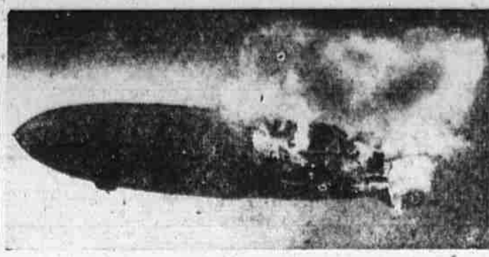
Fire Over Lakehurst Camera catches end of Hindenburg's last ride.
