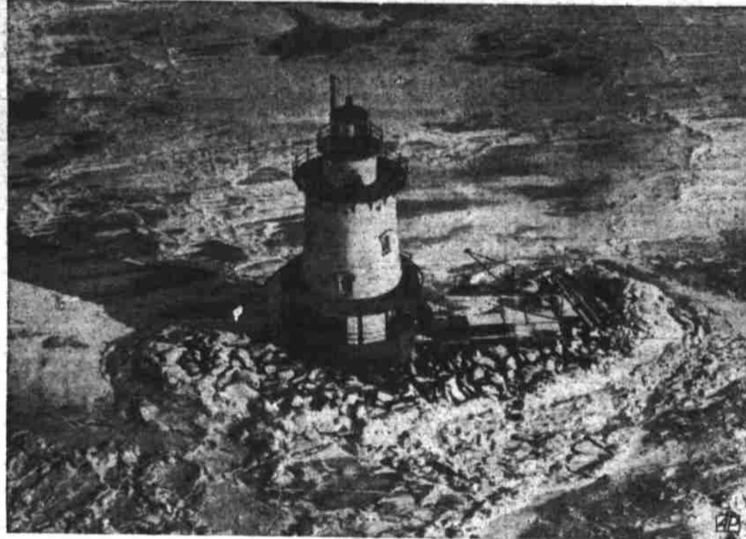
HOUSE IN COLD STORAGE —When zero temperatures swept the Hudson river in upstate New York this river lighthouse south of Bear Mountain presented a desolate, icebound sight.
