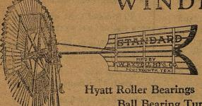
Ball Bearing Turntable Ring Oiling Pitman Self Tightening Wheel
