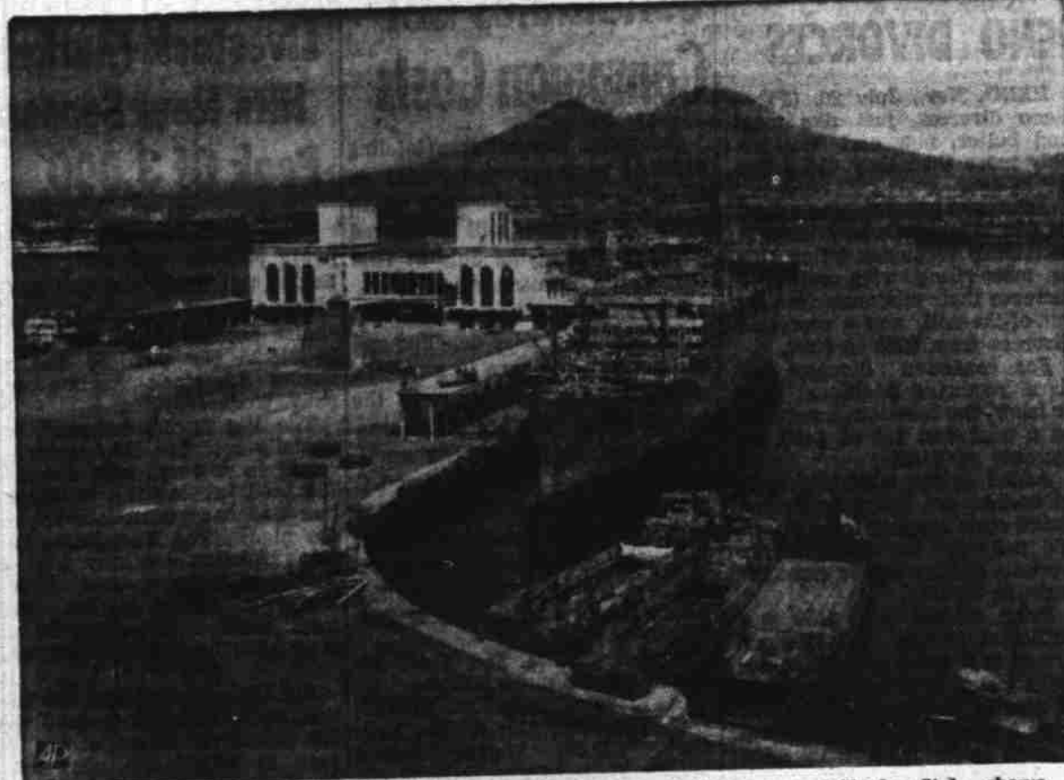
NAPLES HARBOR VIEW—This postwar view of the harbor of Naples, Italy, shows the main pier with the liner Vulcania tied alongside and Mt. Vesuvius in the background.
