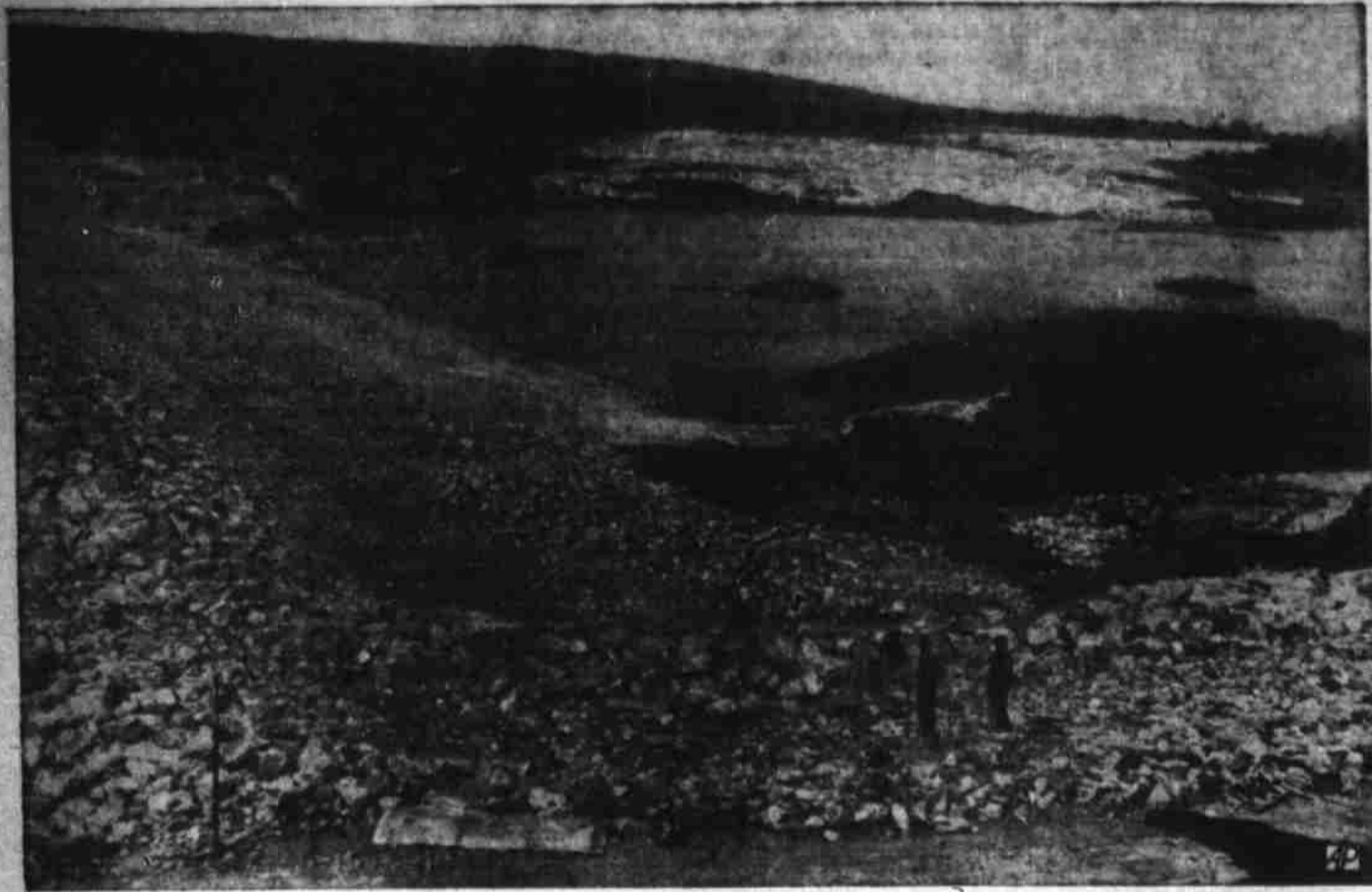
TEARS WERE SHED OVER A TOWN , Enfield, Mass., which after July 1 will be buried under waters of Quabbin reservoir (area at right), being built at estimated cost of $60,000,000 as a metropolitan Boston water supply base. At left is dike of basin in which 400 billion gallons of water 150 feet deep will be stored. The migration of Enfield's 2,000 population began in earnest after the town had its final party in a black and white-draped town hall. There was dancing, beer and regrets as people said farewell to their little community.
