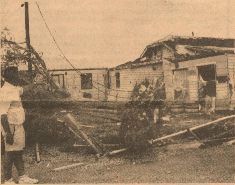
Pictured above is a house located about 5 miles west of Iraan after it was hit by the tornado Friday night.
