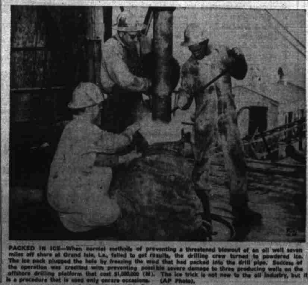
PACKED IN ICE—When normal methods of preventing a threatened blowout of an oil well miser off shore at Grand Isle, La., failed to get results, the drilling crew turned to powdered ice.
