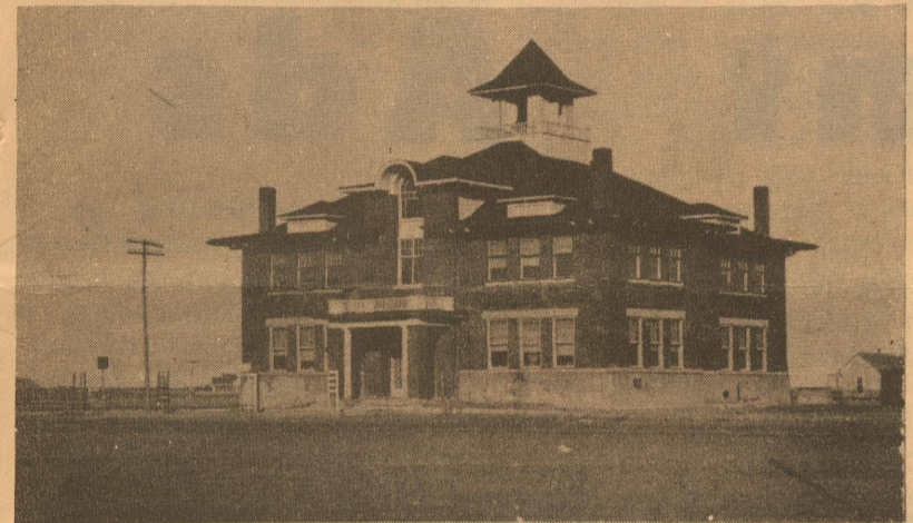
Pictured above is the 1909 Eldorado school building.
