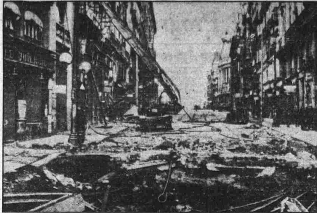
Scores were killed in an underground railway station beneath this Madrid street when an aerial bomb from a Fascist airplane blew this huge hole in the middle of a main Madrid thoroughfare. Hundreds of persons had sought shelter in the station which was wrecked. (Associated Press Photo)
