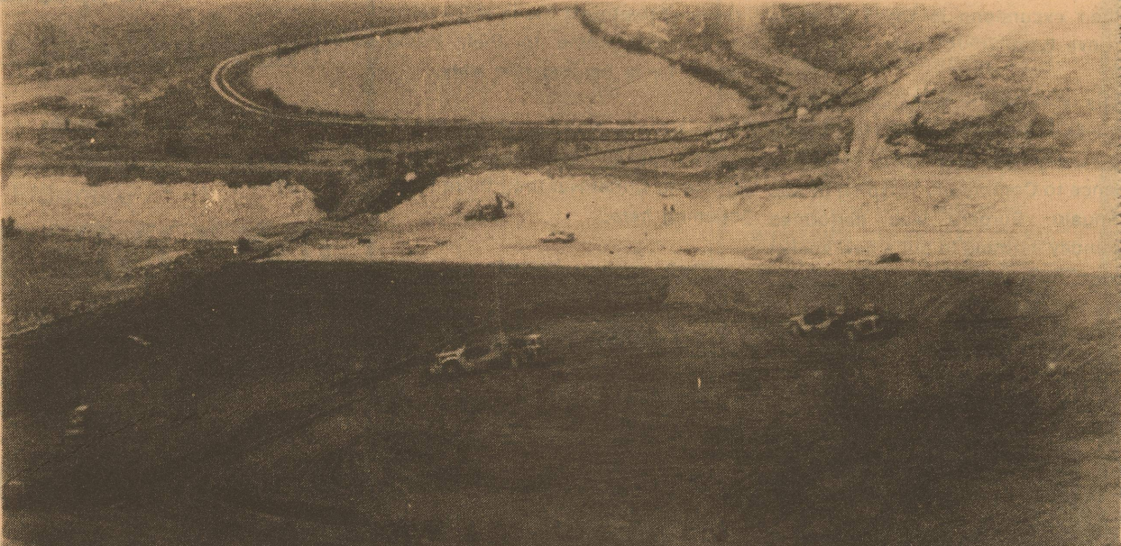
An aerial view of the Waste Water Plant in Eldorado. Courtesy of
