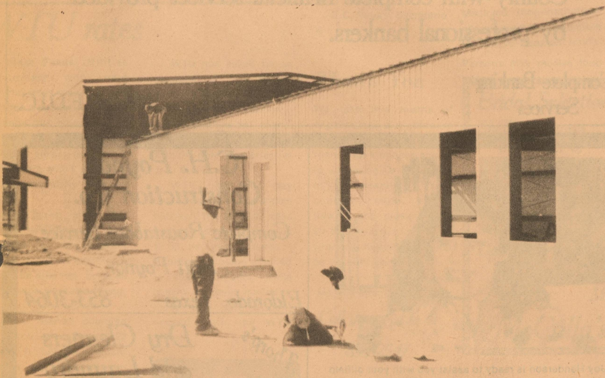
Work on the new Producer's Gas building is progressing on schedule.
