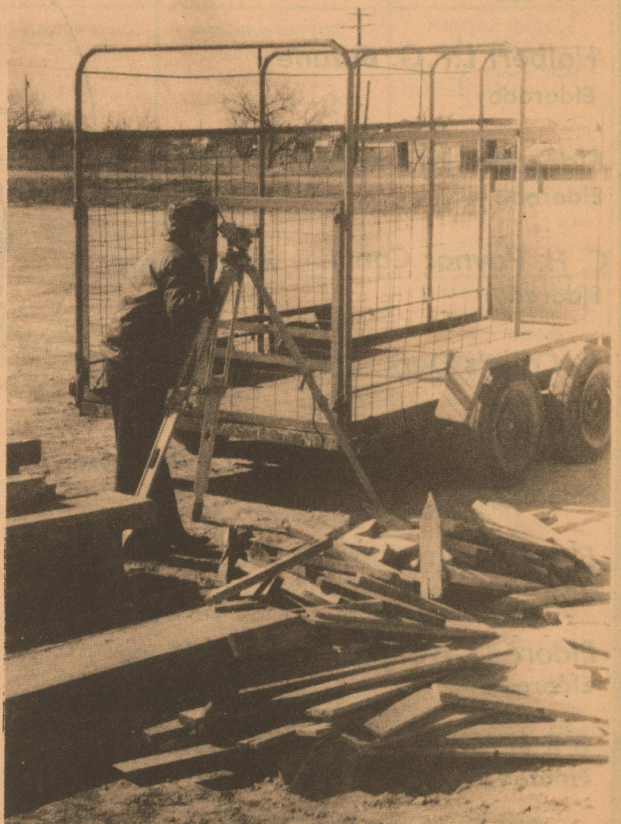
Surveying the property for the future site of Producer's Gas.
