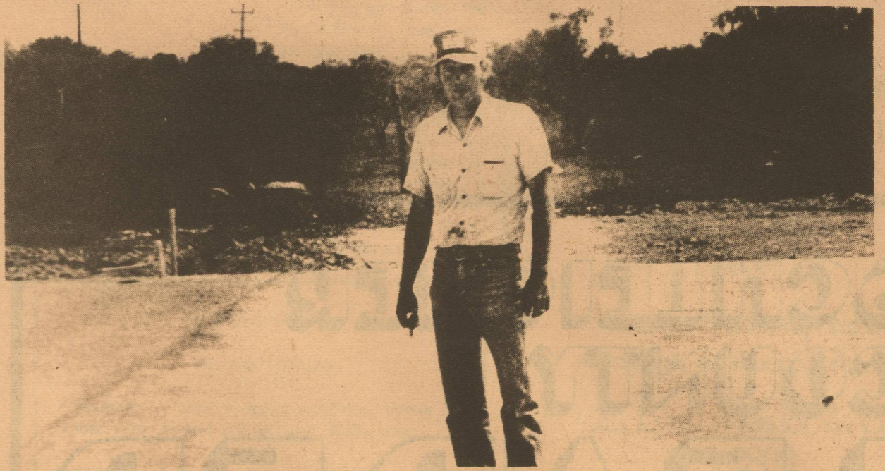
Dan Halbert surveys new sight for Halbert Butane. Building started Mon. 23rd. Mew facilities will house new office, butane tank, and deisel service.
