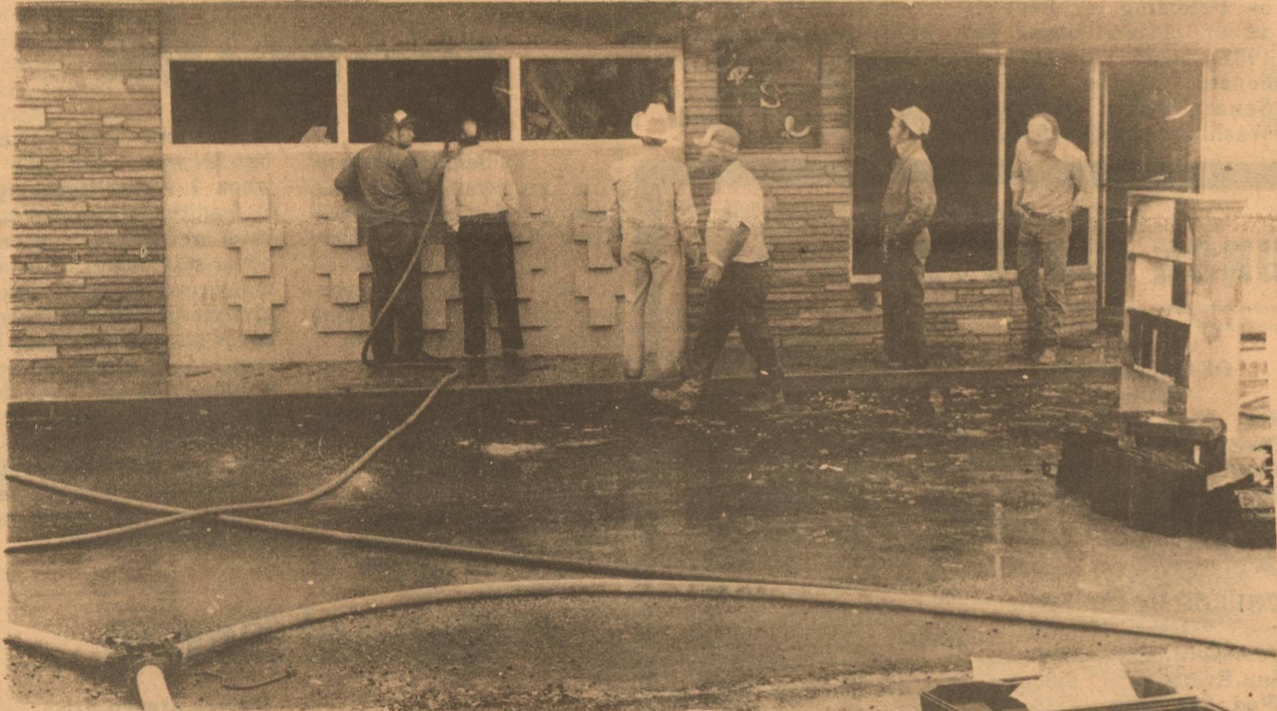
Firemen View Damaged ASCS Building
