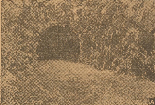
THE CROZET TUNNEL —This 4,273 foot tunnel, completed in 1858, represents the culmination of civil engineering technology when based on manual drilling methods. It was the longest railroad tunnel in the United States and was designed and built by Claude Crozet.
