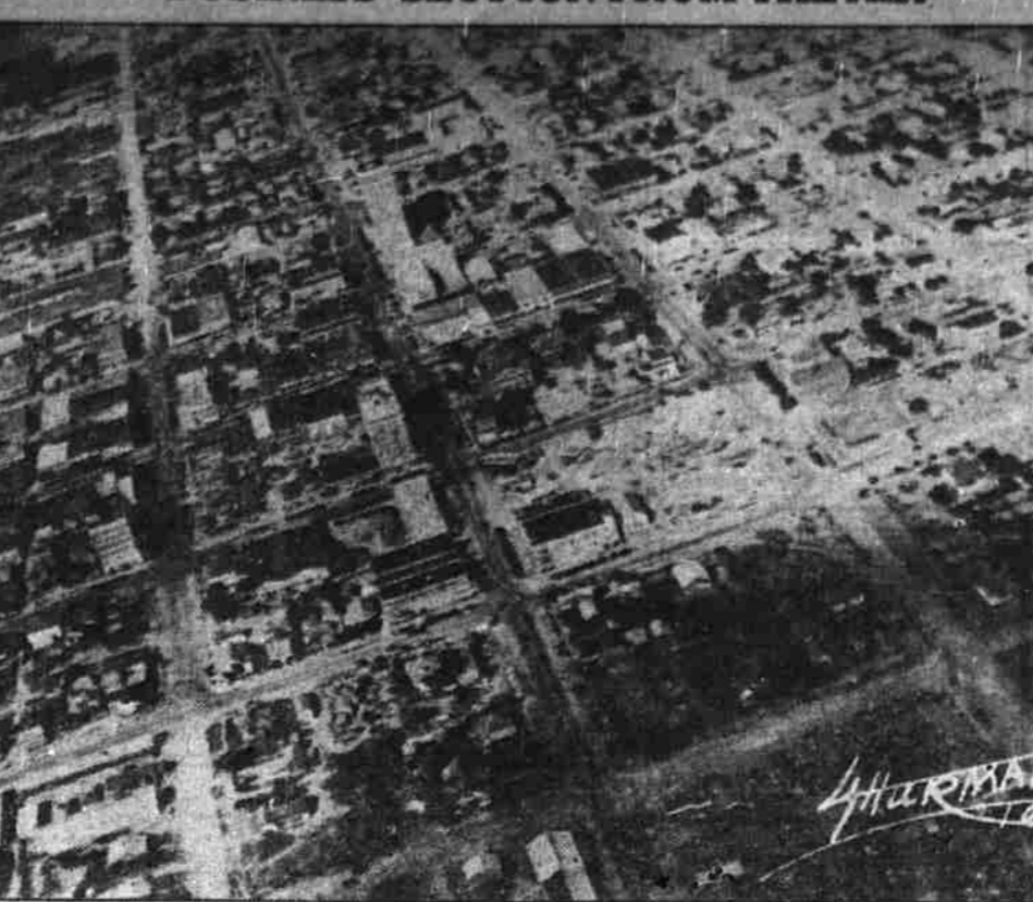
Here is another view of a series of pictures of Big Spring and vicinity taken from the air. This is a picture of the main business area along the Broadway of America highway. Big Spring's tallest building, the Settles Hotel, may be seen in the background. The Crawford Hotel is shown about the middle of the picture.
