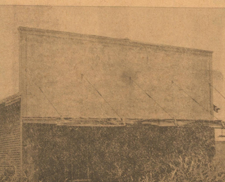
Many years ago Wm. Cameron lumber firm used this orange building on South Main. It was subsequently locked up and unused and now all the windows are broken out and the roof is deteriorating. Shoulder-high weeds surround the structure.
