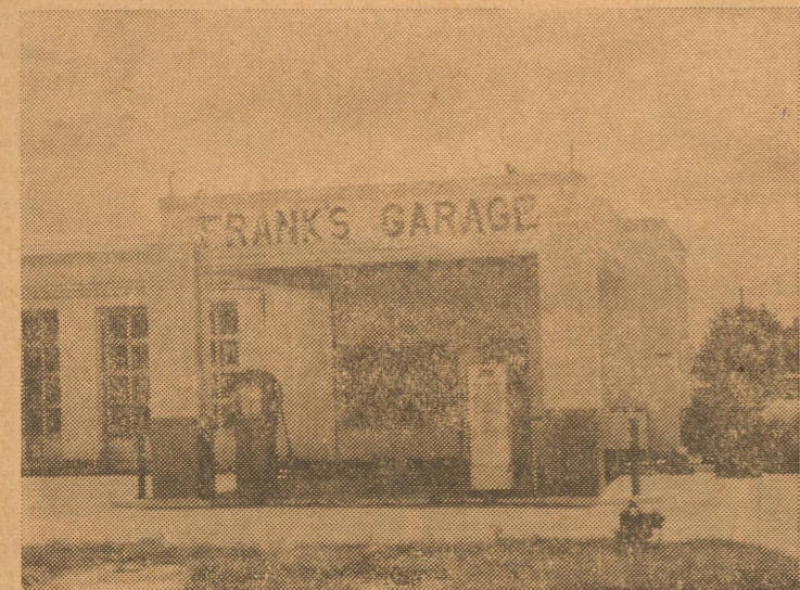
Laborers with shovels dug the pits for the gasoline storage tanks for this garage station, about 40 years ago. The most recent enterprise was "Frank's Garage" and the structure sustained some fire damage at one time. It is used now for storage.
