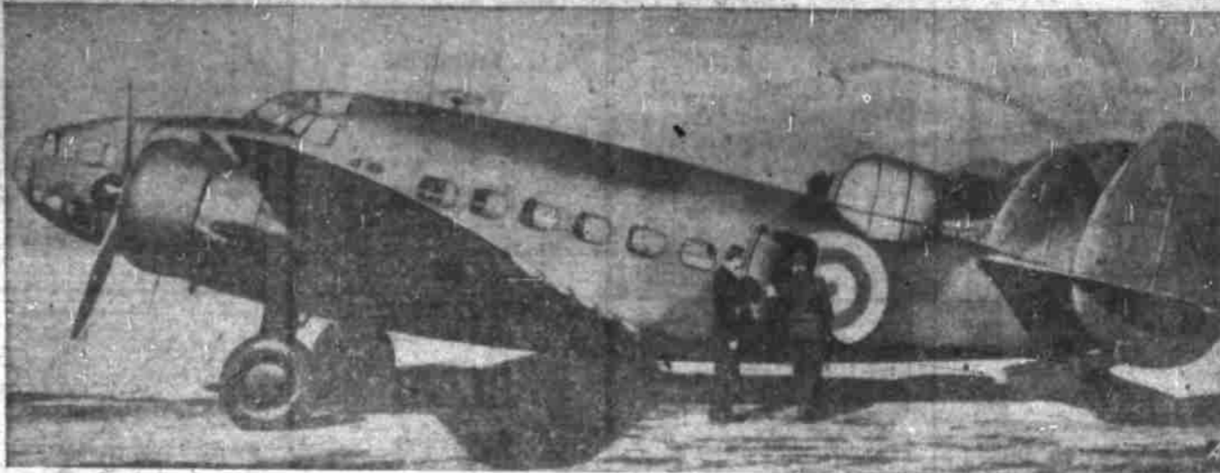
BRITAIN'S FIRST AMERICAN-BUILT BOMBER (above), given tests at Burbank, Cal., is a Lockheed B-14 carrying a crew of four. It is painted in the camouflage coloring of Britain's Royal Air Force and has gun openings on the fuselage at rear and in the nose.
