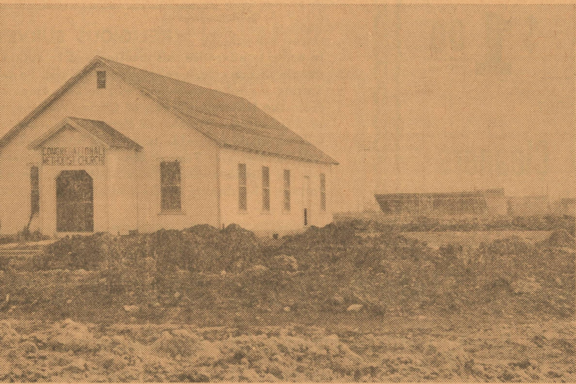
Church Building Still Remains To Be Moved
