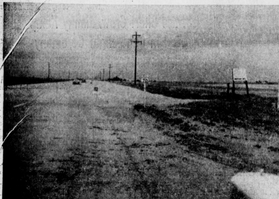
U.S. 70 FLOODED, TOO - Water snaked across U.S. 70 in several places between here and Earth after this past week's downpours. This shot was made 10 miles east of Muleshoe at the Bailey-Lamb county lines. The water stretched across the highway for more than half a mile.
